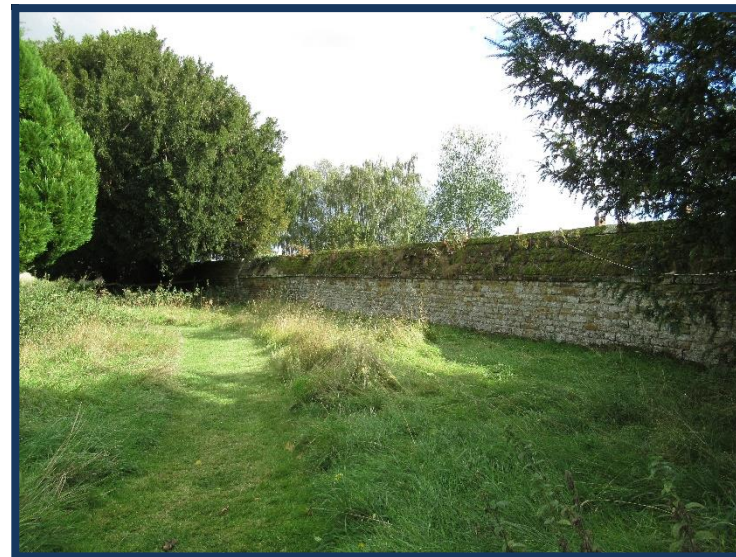
Figure 32: Wall of the 16 th century walled garden
