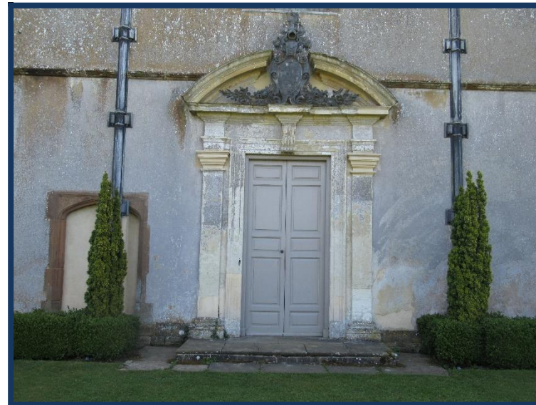
Figure 28: 18 th century entrance in northwest elevation
