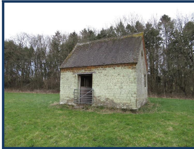
Figure 42: Barn northwest of Park Cottage
